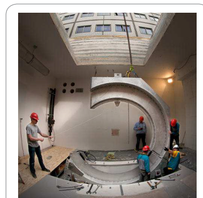
Building of the MR-Linac system at UMCU
